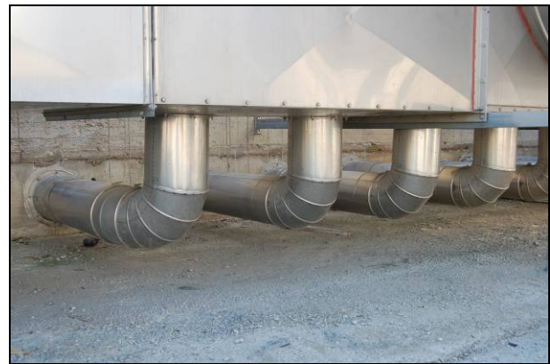
Fig. 2 Detail of the air inlet tubes
