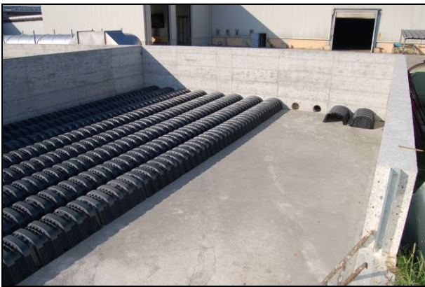
Fig. 1 Installation of Drening
