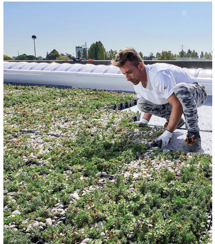
Laying system Complete
