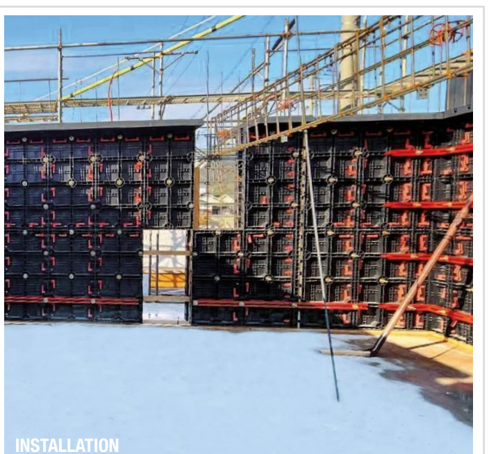
Geotub construction site for railway footbridge Aarsleff, Denmark
