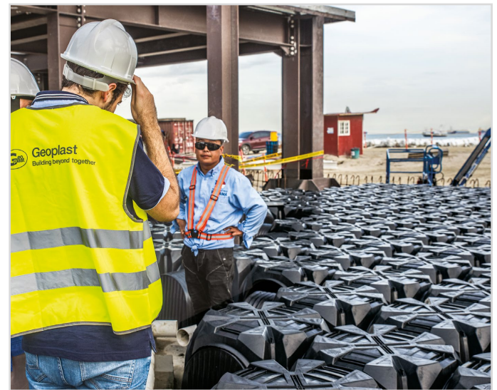
Modulo on-site installation
