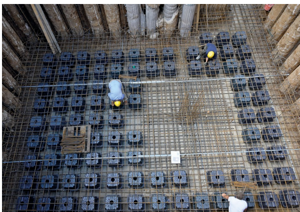
COMMERCIAL-RESIDENTIAL BUILDING St. Cross Square - Tivoli, ITALY Complete building and slab design.
